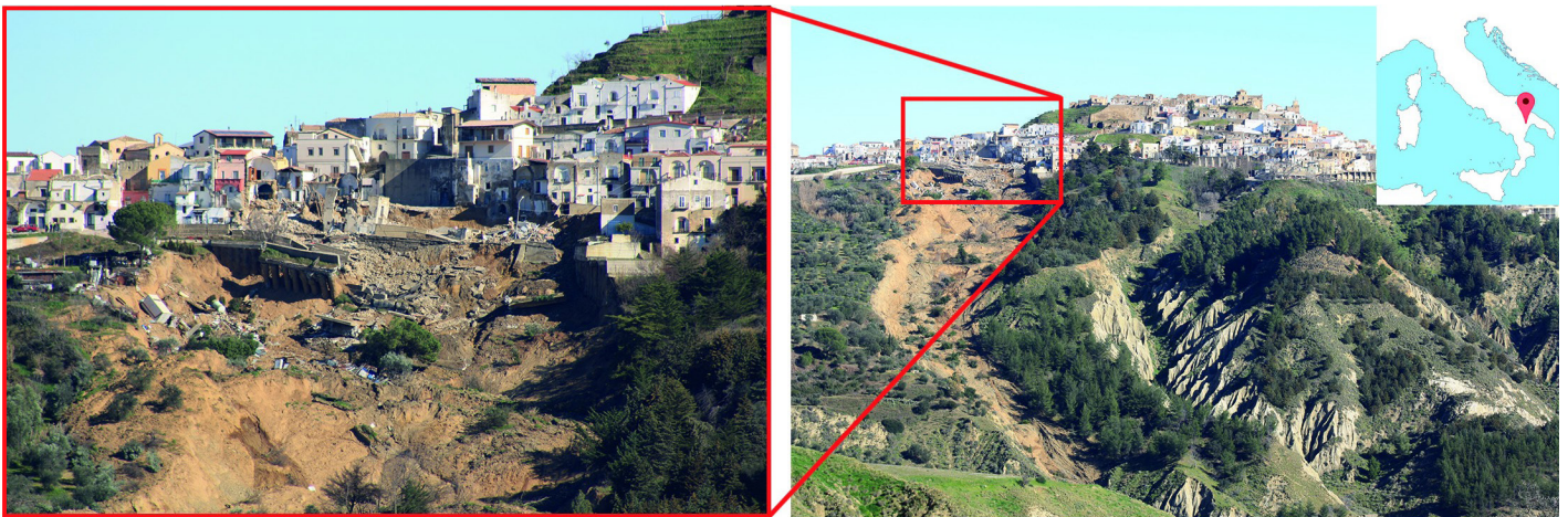
Fig. 1 - View and location of the study area. On the left: collapsed road, damaged and collapsed buildings and rubble accumulations on the upper part of the slope. On the right: view of the landslide slope.
